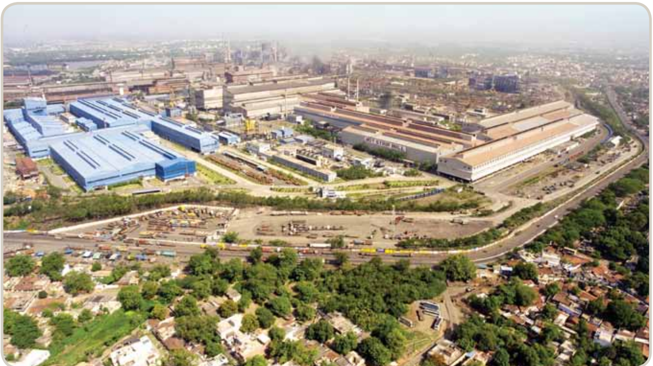
Pan-view of facility in Jamshedpur, India
