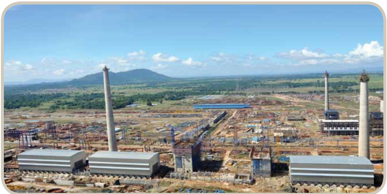
Kalinganagar project speeding towards completion, Odisha, India
