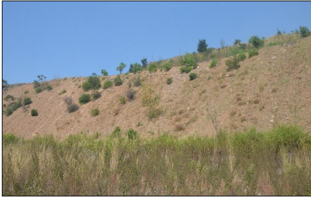
Top Soil spreading on dump for plantation
