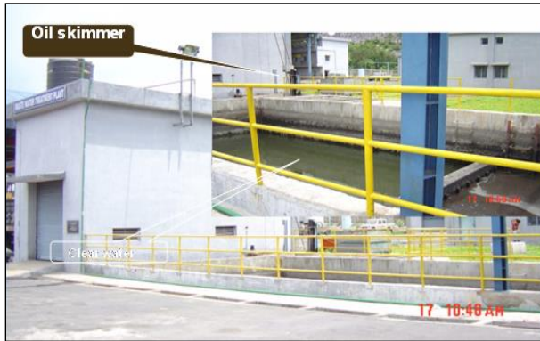
Oil & Grease trap at mines
