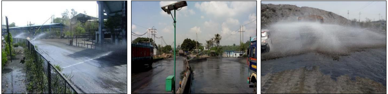
Use of fixed & mobile water sprinklers
