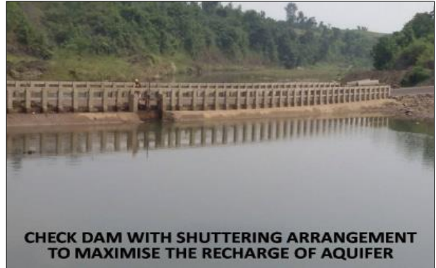
Check Dam to increase ground water recharge
