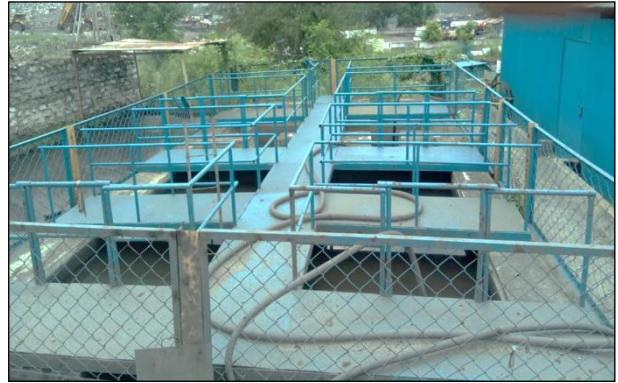
Oil & Grease trap at mines
