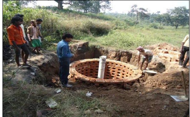
Artificial ground water recharge pit (Bore well) in Birhor village
