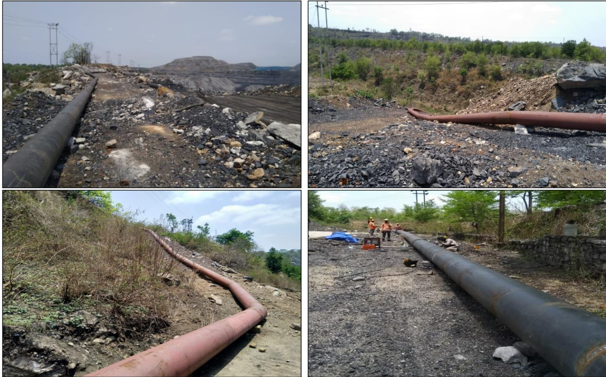
Pipeline installation from active quarry pit to abandoned mine pit
