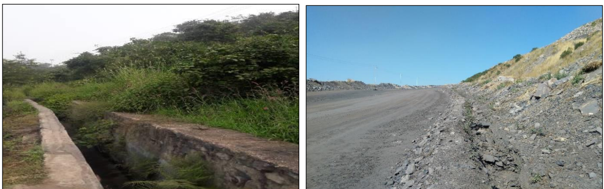
Catch Drains at the toe of dumps
