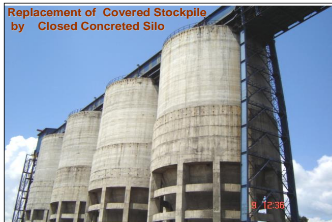
Concrete silos for material storage
