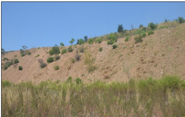
Soil & grass Spreading on dump slope
