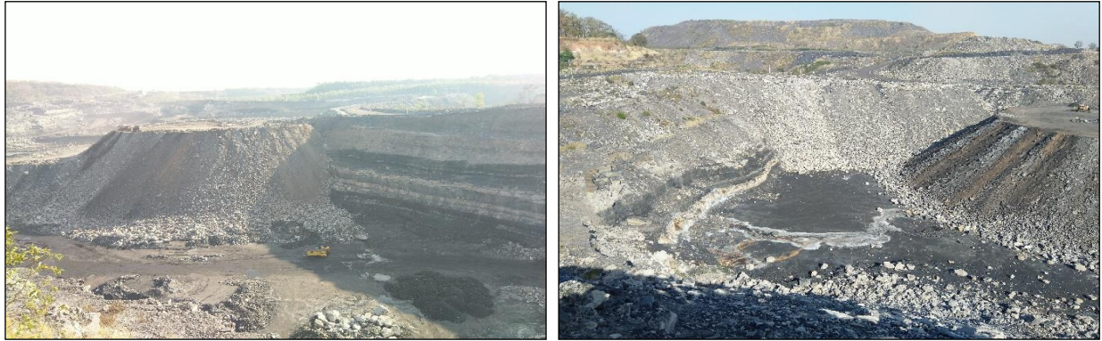
Back filling of quarry by Over Burden
