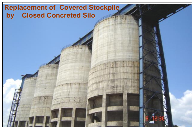
Concrete silos for material storage
