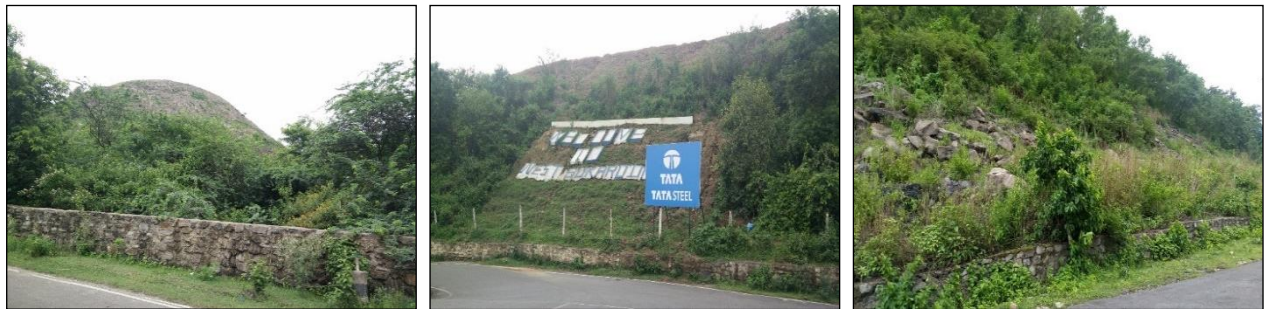
Toe walls on dumps
