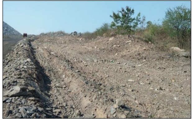
Maintained catch drain of Top Soil Dump
