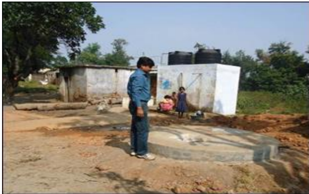
Artificial ground water recharge pit (Bore well) in Birhor village
