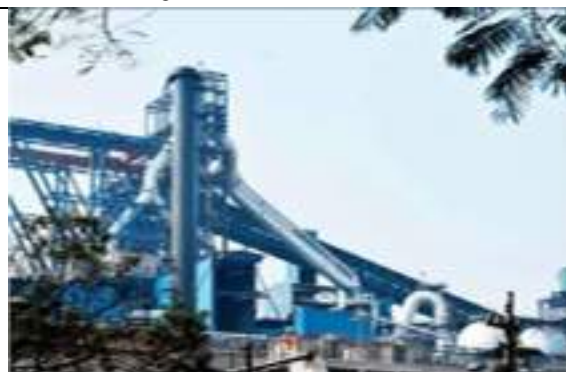
High Efficiency BF with high Top Pressure, Stove Waste Heat Recovery, TRT, Cast House Slag Granulation
