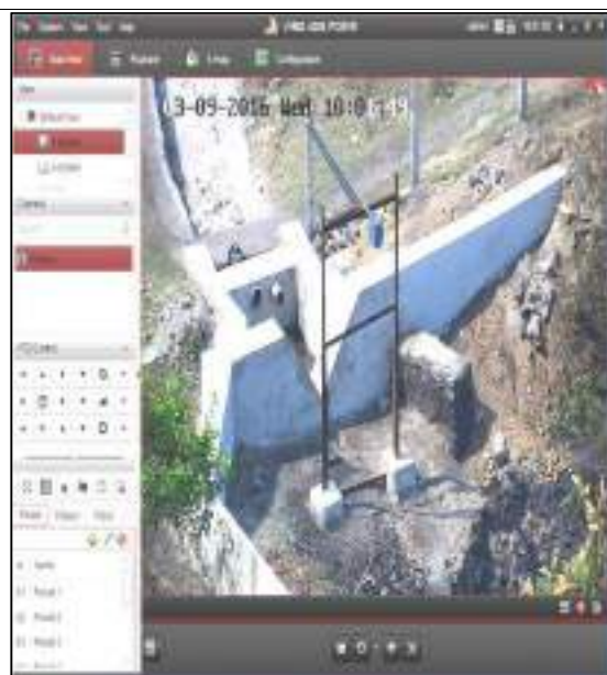
Effluent Analyzers & Monitoring
