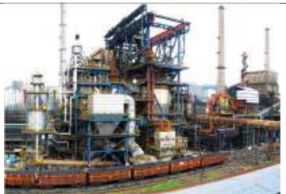
Waste Heat Recovery in Coke Dry Quenching
