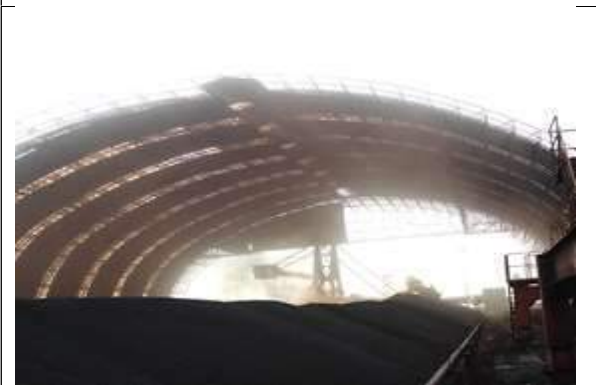
Covered Shed for Coal and Pellet
