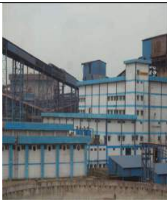
Reverse Osmosis Building
