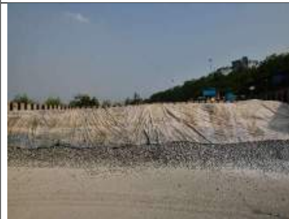
Open Steam Aging plant for LD Slag
