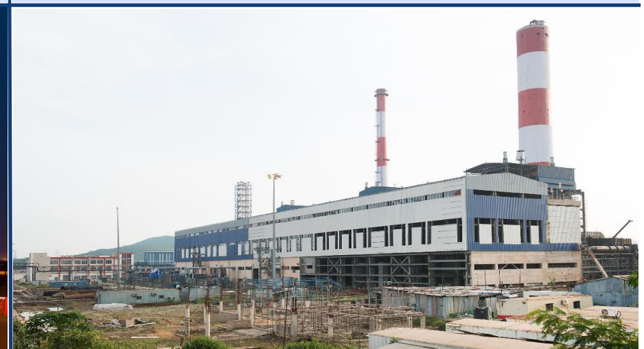
Backside view of the power plant
