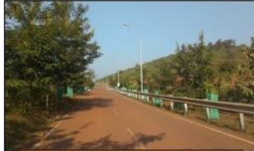
Mine road side plantation
