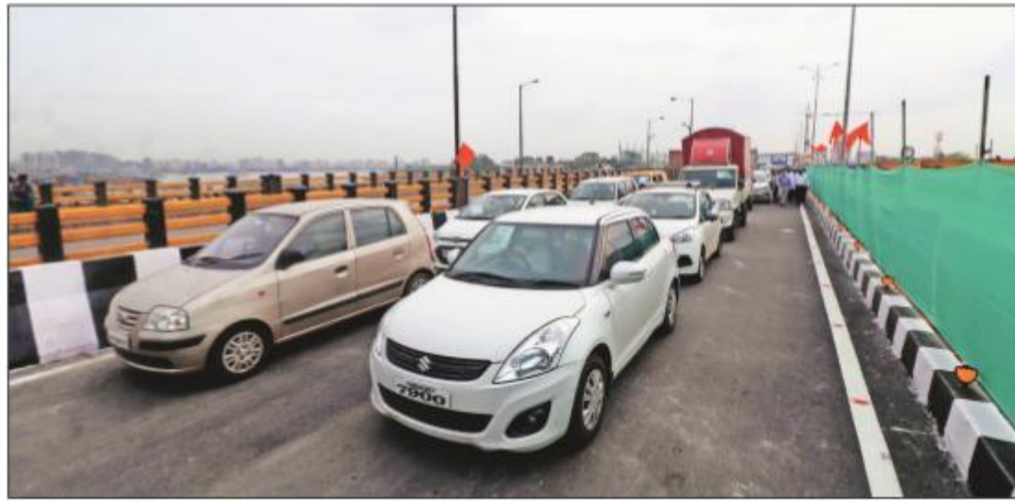
The Kalyan Durgadi bridge was opened on Monday. Deepak Joshi
