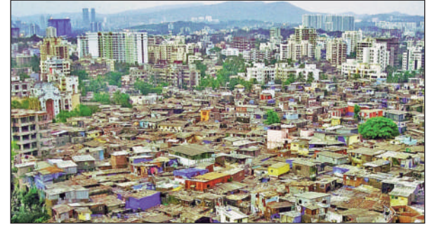
The civic body said most slums violate guidelines by adding more floors
