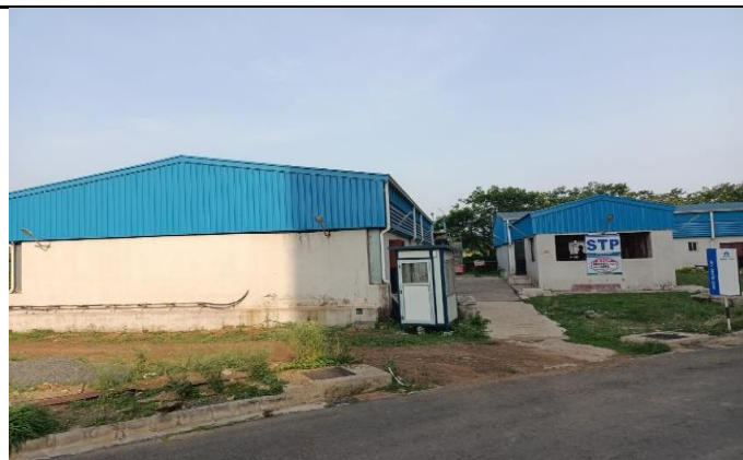
Sewage Treatment Plant in Operation
