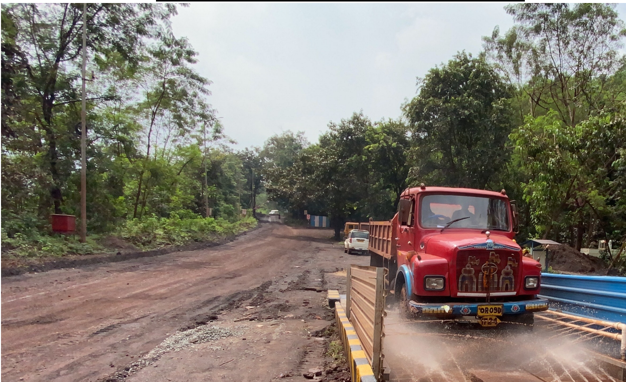
Fig.1 Automatic Wheel Wash Facility @ Bamebari Iron & Mn Mine
