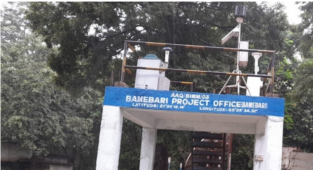
Fig.3 AAQ Station Near Project Office (Bamebari Iron & Mn Mine)
