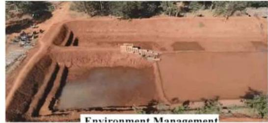
**Surface Runoff Management: Network of Garland Drains, Toe Wall & Rain Pass**
