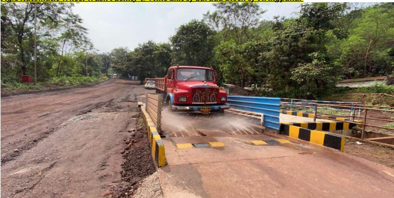
**Fig.2 Automatic Wheel Wash Facility @ Guruda Block of Tiringpahar**
