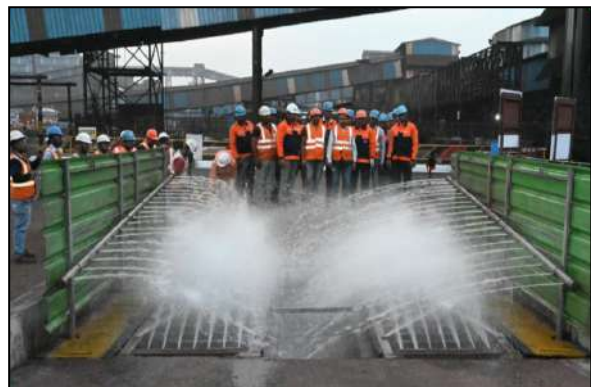
Wheel washing system at RMHS
