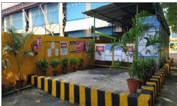
Hazardous waste storage shed at HSM Water Complex
