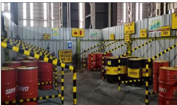
Hazardous waste storage shed at BOF
