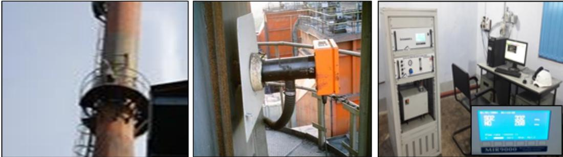
Continuous Emission Monitoring for Power House for PM, Sox & NO<sub>x</sub> data
