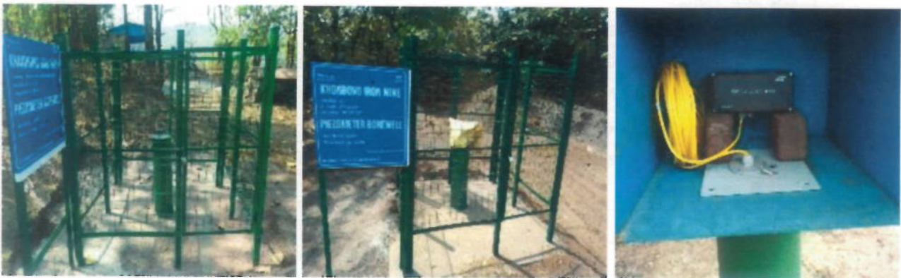
Piezometer (STP and Manganese) with digital recorder
