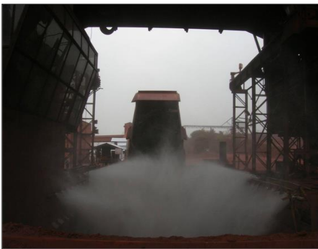
Water Jet System at Unloading Point
