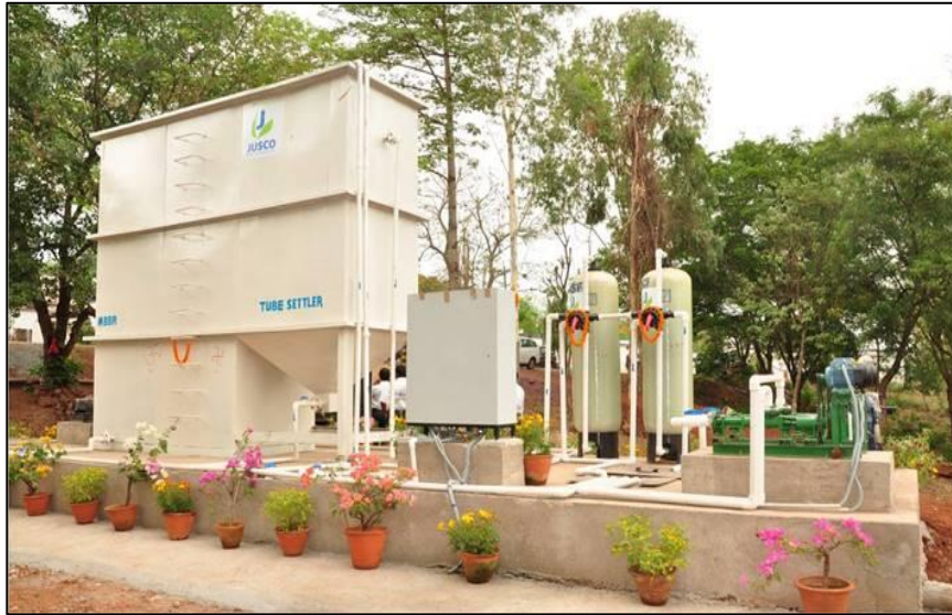
Sewage Treatment Plant
