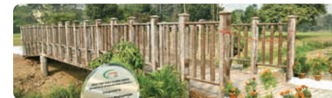
Bridge at Golmuri Golf Club in Jamshepdur made of Fibre Reinforced Polymer (FRP) Composites
