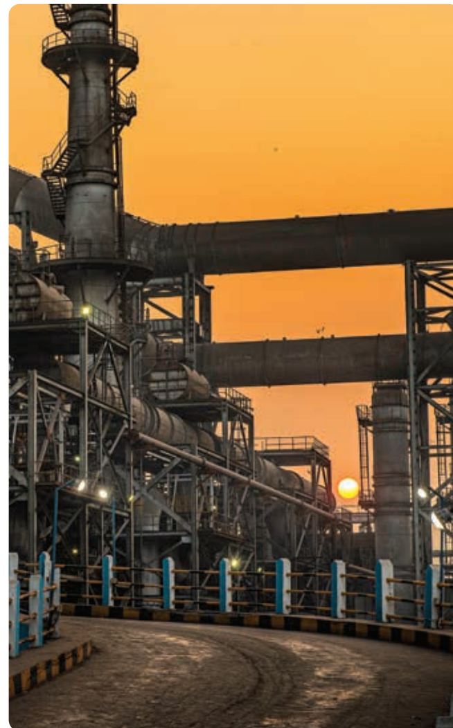
Blast Furnace, Tata Steel Meramandali Works
