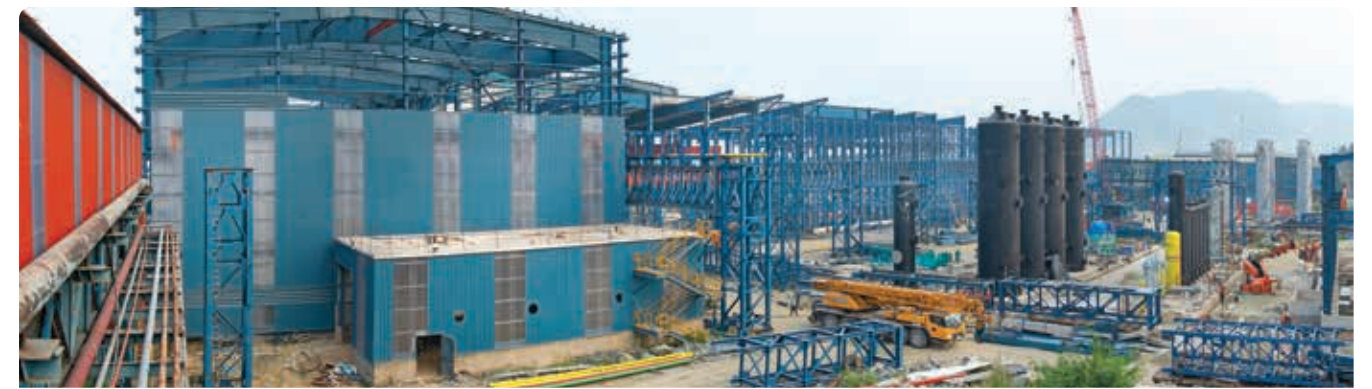
5 MnTPA expansion work underway at Tata Steel Kalinganagar
