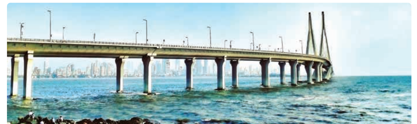
Bandra Worli Sea Link, Mumbai (Tata Steel's state-of-the-art durable LRPC strands and Tisco reinforcement bars were used in the construction)
