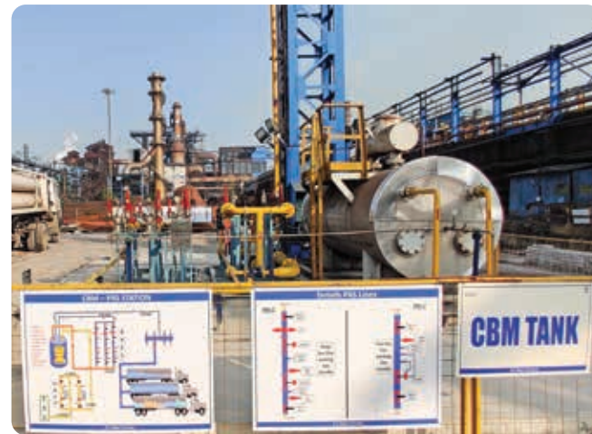
Plant trial of continuous injection of Coal Bed Methane gas in blast furnace. The technology is expected to reduce CO 2 emission by reducing coke rate by 10 kg/thm, which will be equivalent to reducing 33 kg of CO 2 per tonne of crude steel
