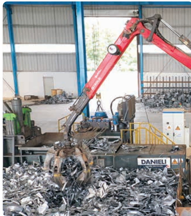
Steel Scrap Recycling Plant at Rohtak, Haryana
