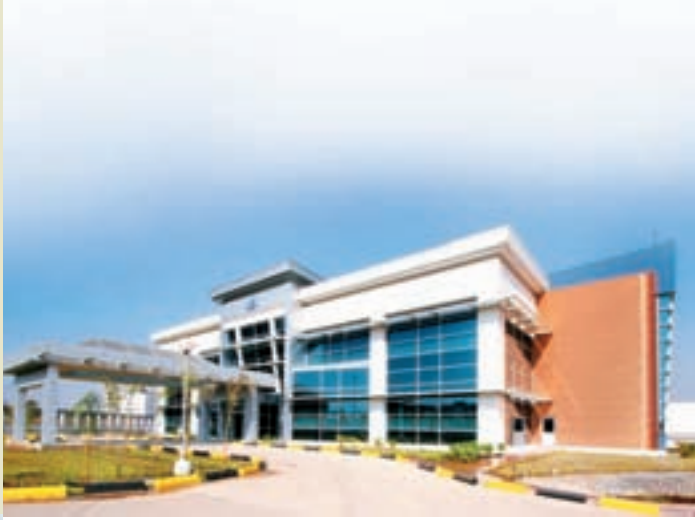
Tata BlueScope Steel Limited has started operations with its first pre-engineered building manufacturing unit in Pune.
