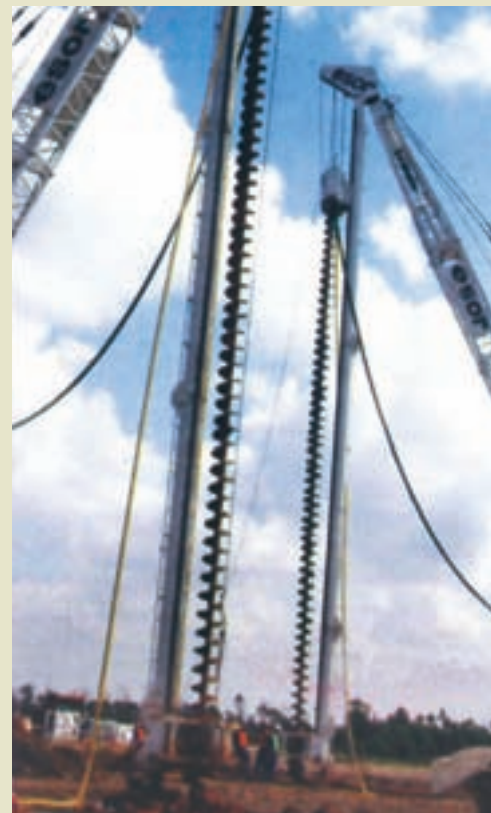
Construction work has commenced at Richards Bay
