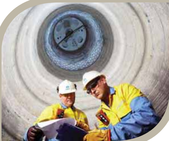
Inside the shell of the new No. 4 Blast Furnace at Port Talbot
