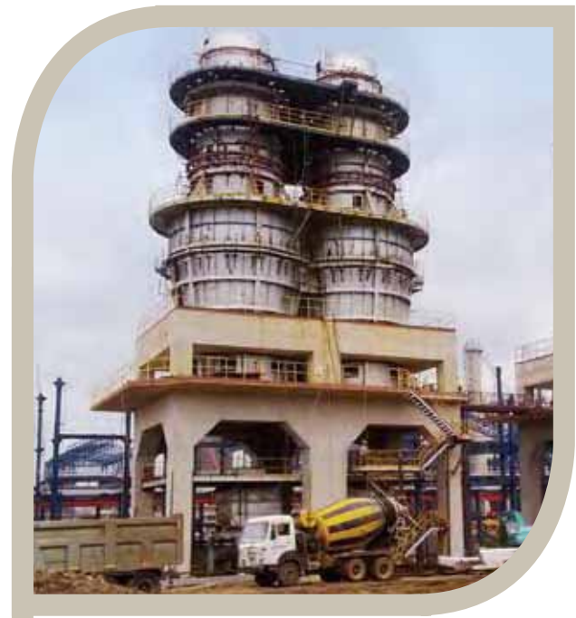
Greenfield project – Kiln 2, Odisha, India
