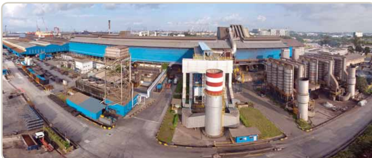
Baghouse facility at NatSteel, Singapore
