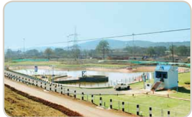
Water Harvesting Park, Joda, Odisha
