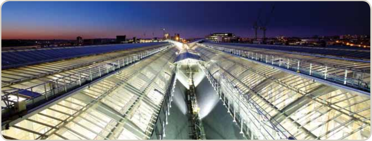
Tata Steel used in the redevelopment of King's Cross Station in London, Europe
