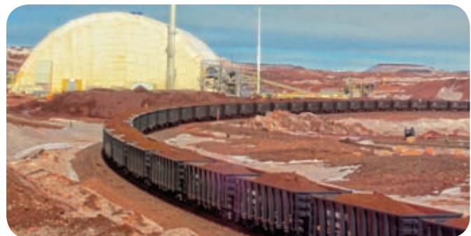
Processing facilities and Rail Loop
