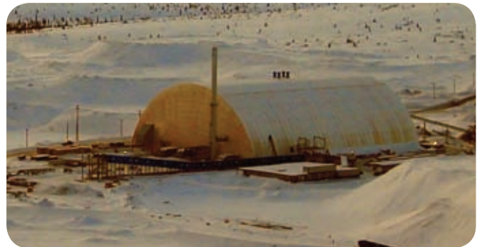
Dome - Processing facilities
