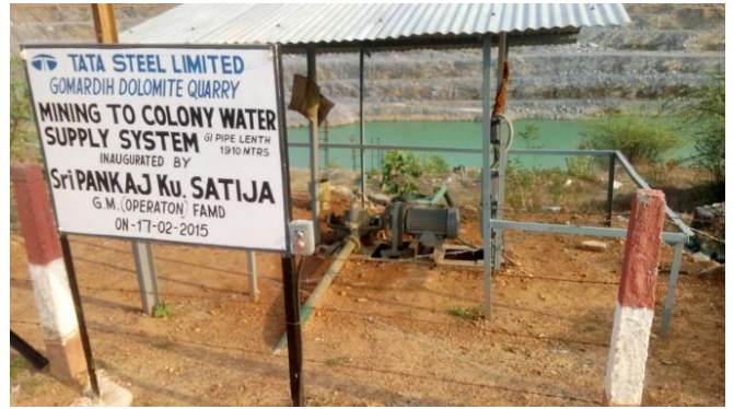
ARRANGEMENTS FOR PUMPING AND TREATMENT OF ACCUMULATED RAIN WATER OF THE QUARRY
