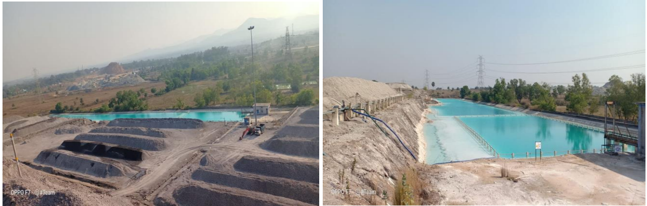
Rainwater Harvesting Pond
