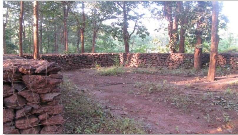
Check Dam for Surface Runoff Management
