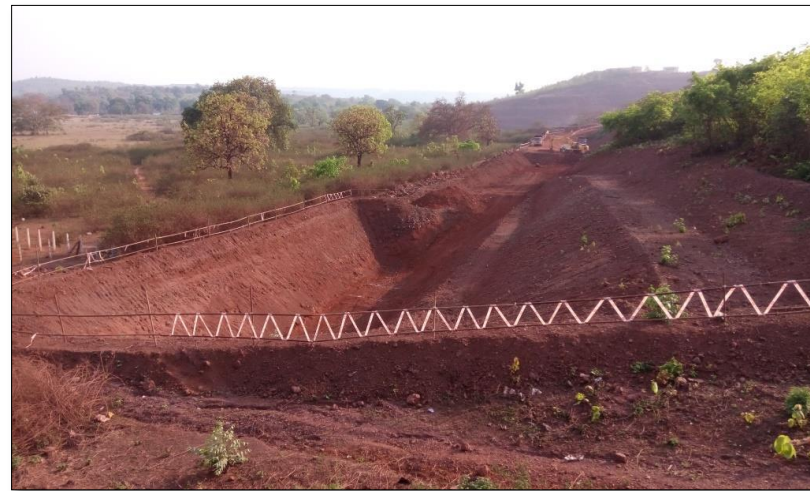
Settling Pit for Surface Runoff Management
