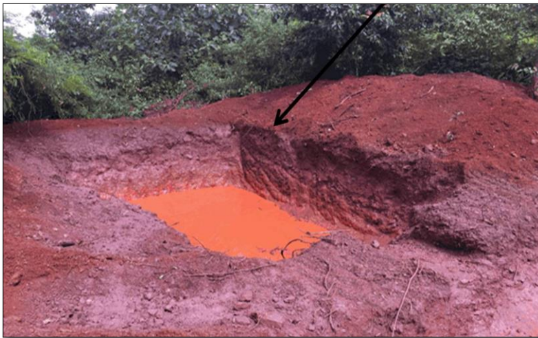
Settling Pit for Surface Runoff Management
