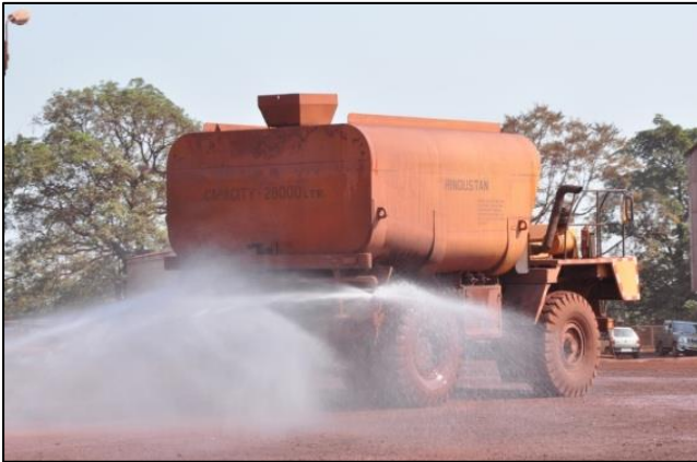
Mobile Water Sprinkling
