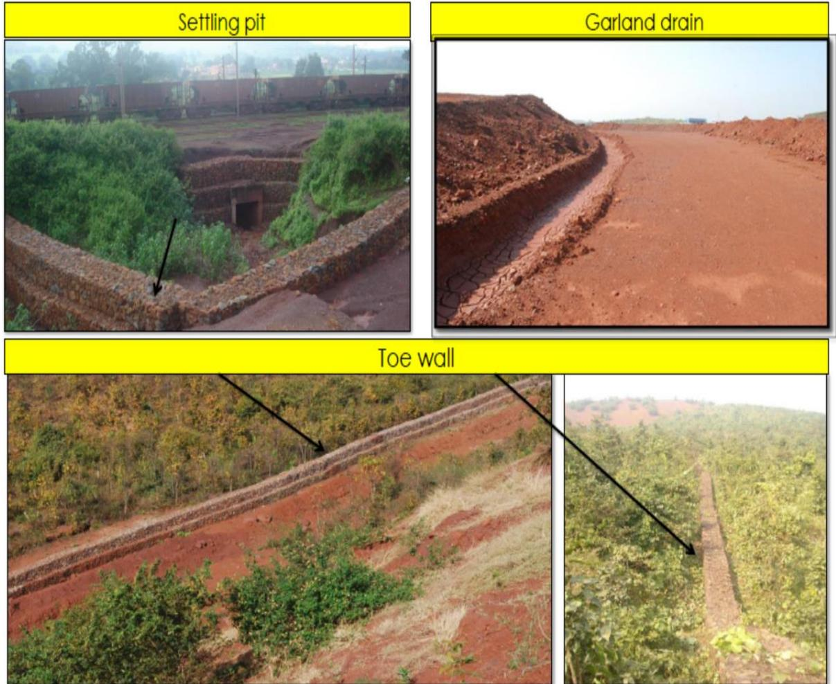
**Garland Drains, Toe Walls, Settling Pits: JEIM**
