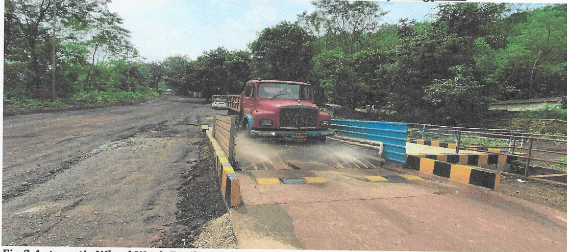
Fig.2 Automatic Wheel Wash Facility @ Guruda Block of Tiringpahar
