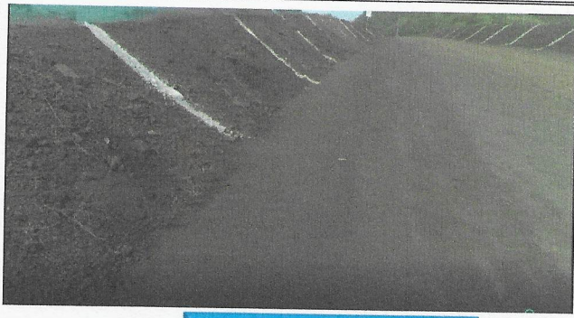
Mine Haul Road
