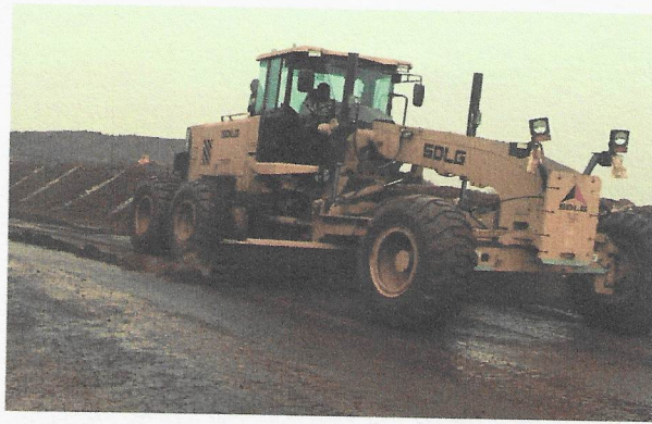
Grader for Haul Road
