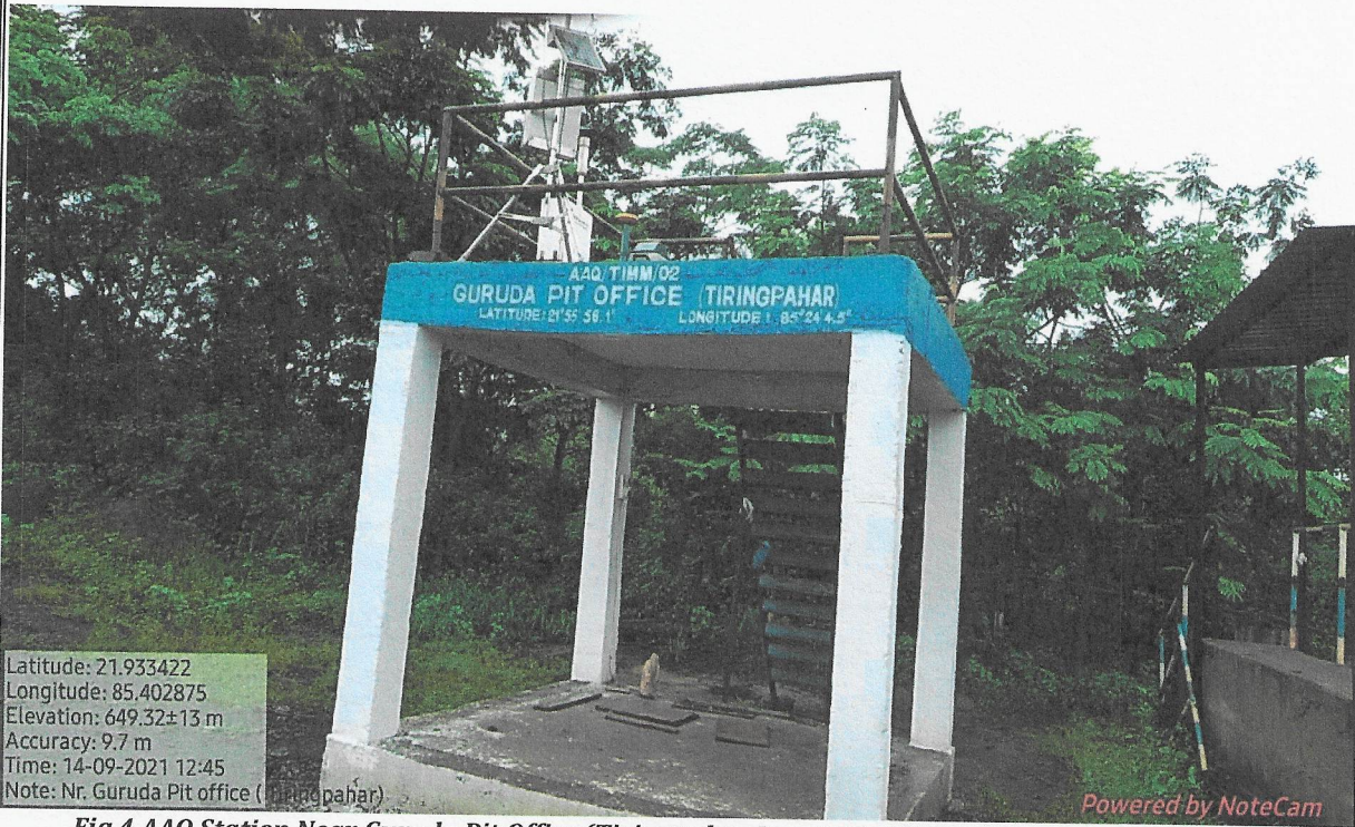
Fig.4 AAQ Station Near Guruda Pit Office (Tiringpahar Iron & Mn Mine)
