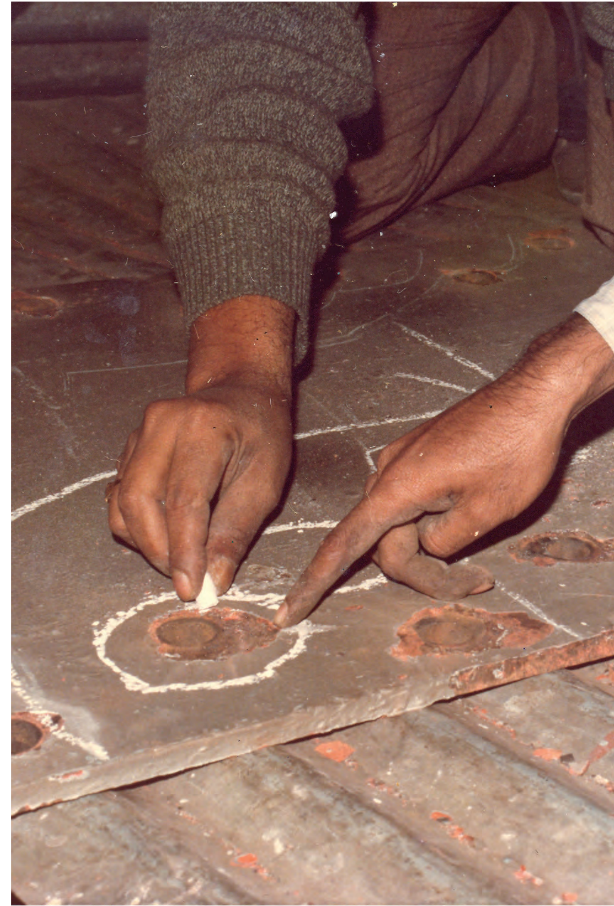
Inspection at the soffit of the top chord of the suspension span
