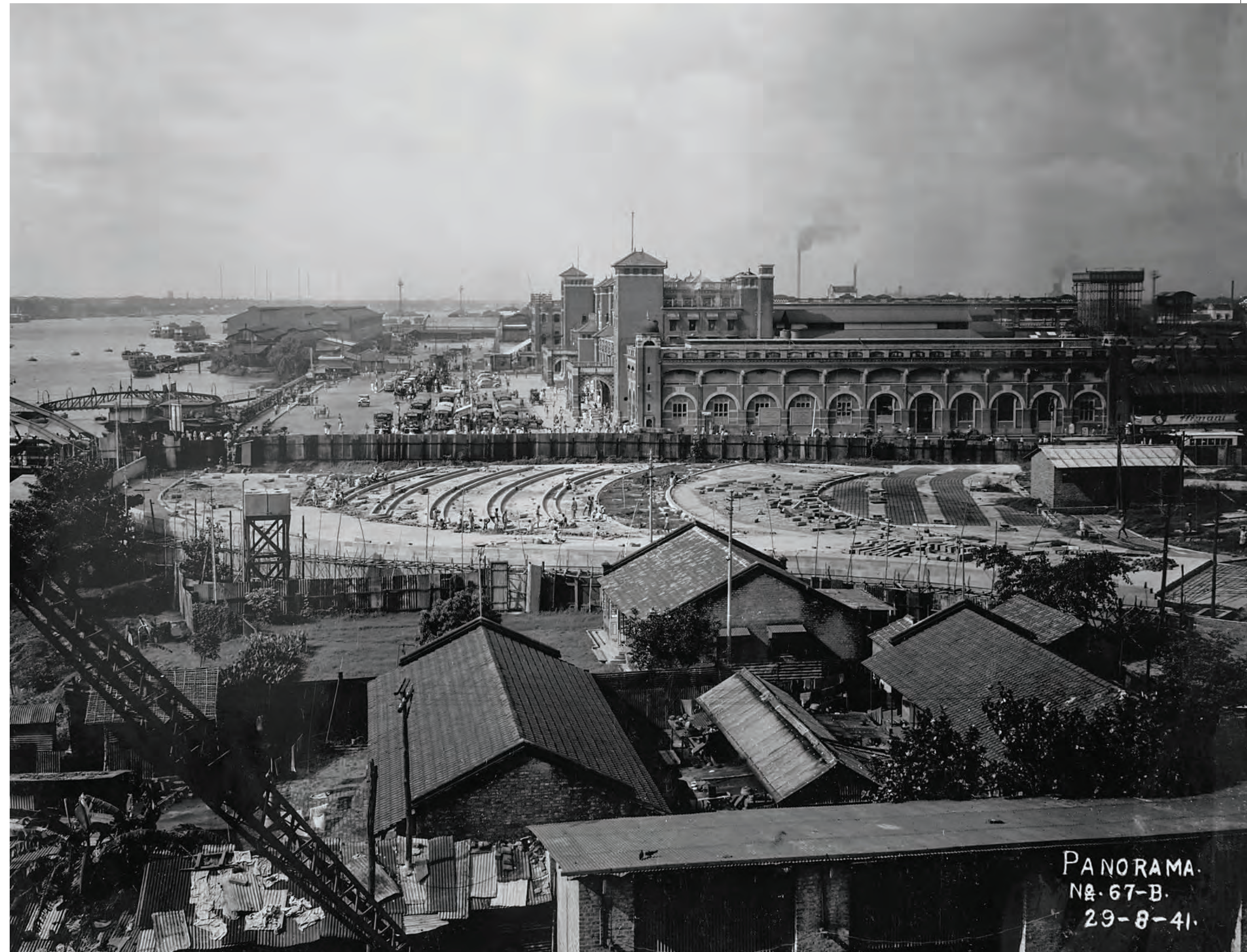
Panoramic view of the site, station end
