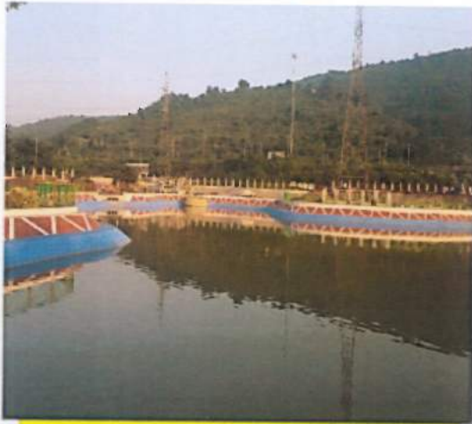
New Rain water Harvesting structure
