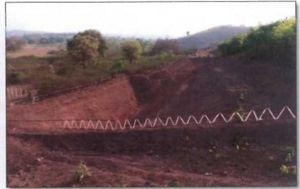
Settling Pit for Surface Runoff Management
