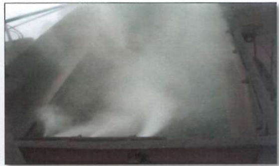
Dry Fog at Crushing & Screening Plant
