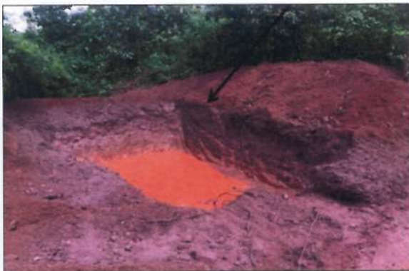
Settling Pit for Surface Runoff Management
