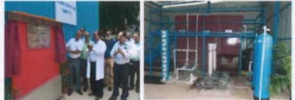
10 KLD ETP at TATA Steel Hospital, Noamundi
