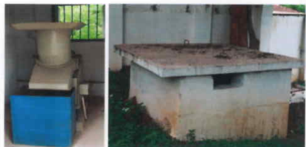
Plastic shredder, deep burial-ash disposal pit at Hospital
