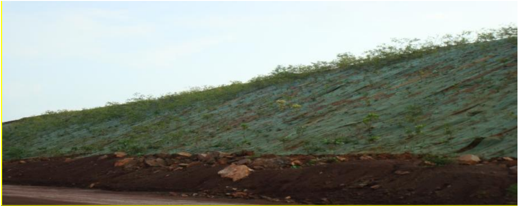
Vetiver Plantation and Coir Matting
