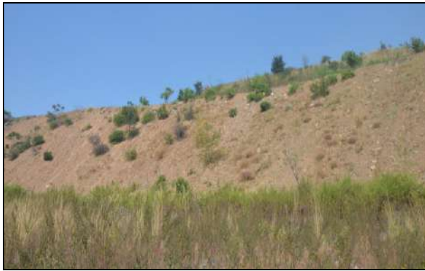
Soil & grass Spreading on dump slope
