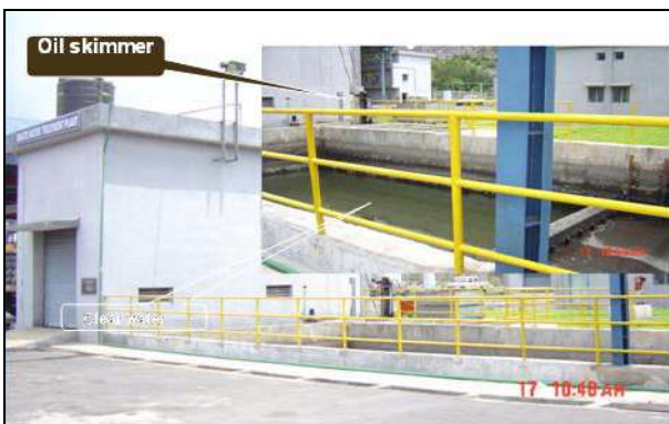
Oil & Grease trap at mines
