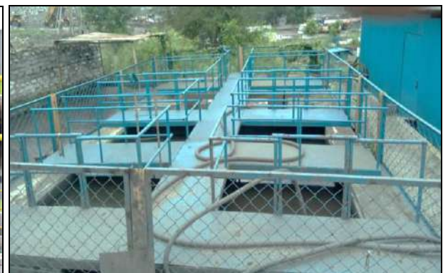
Oil & Grease trap at mines
