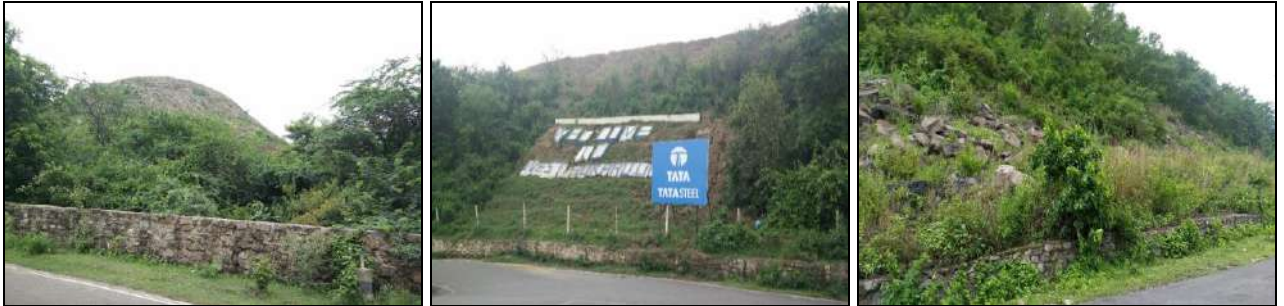
Toe walls on dumps
