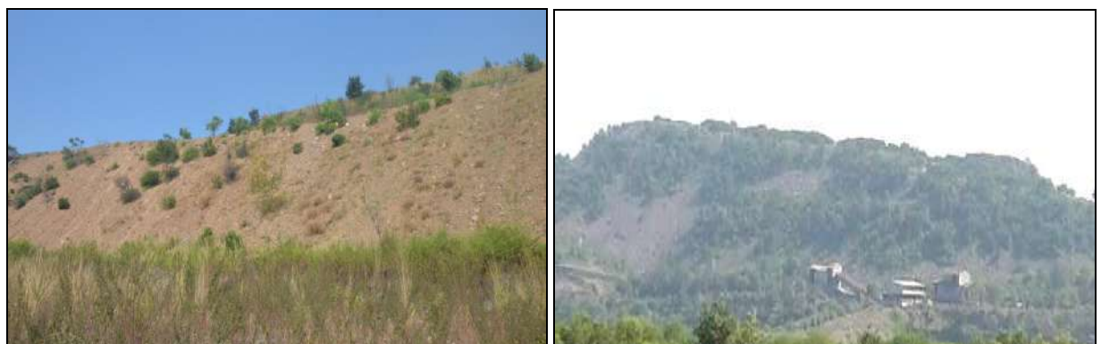
Soil & grass Spreading on dump slope
