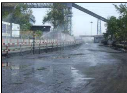
Fixed and mobile water suppression system
