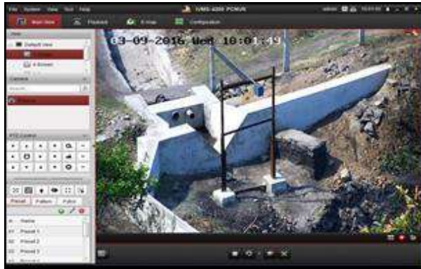
Live web camera footage installed at discharge point
