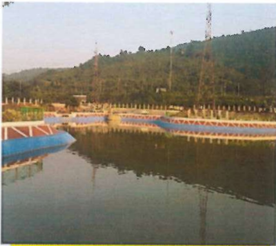
New Rain water Harvesting structure
