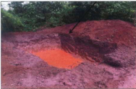
Settling Pit for Surface Runoff Management
