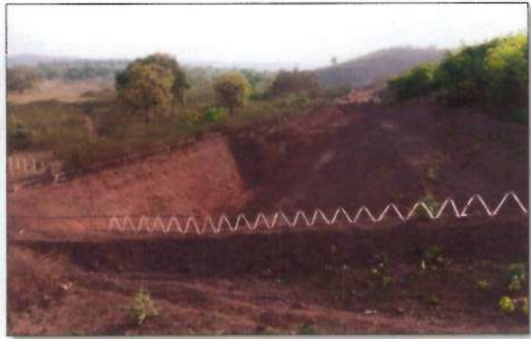
Settling Pit for Surface Runoff Management
