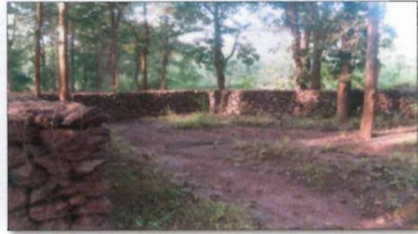
Check Dam for Surface Runoff Management
