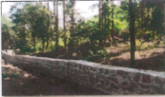
Toe Walls at Dumps
