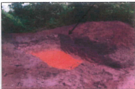
Settling Pit for Surface Runoff Management
