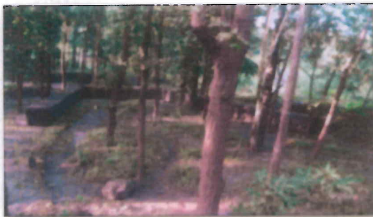
Check Dam for Surface Runoff Management
