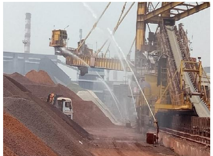
Water sprinkler at raw material yard
