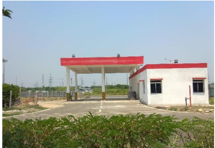
Second Fire Station at TSK
