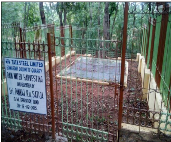
RECHARGE PIT OF ROOF TOP RAIN WATER HARVESTING STRUCTURE OF GUEST HOUSE OF GOMARDIH
