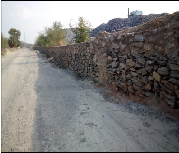
MINERAL STACKYARD TOE WALL
